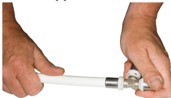
*Insertion and twisting of the deburred plastic pipe.*
