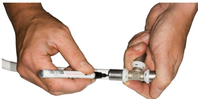
The insertion depth is marked with a pen.
