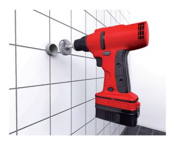
23. The wallbox is cut down to approximately 5 mm from the completed wall with **LK Wall Box Cutter UNI** (Article no 187 64 94).
