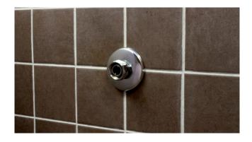
For assembly of tap mixer in accordance with Swedish standards, **LK Connection coupling M26** (Article no. 187 05 47) should be assembled. The length of the connection should be adjusted and the thread joint against the angle fitting should be sealed with, for example, flax and thread paste. Tightening is done with a combination wrench.
